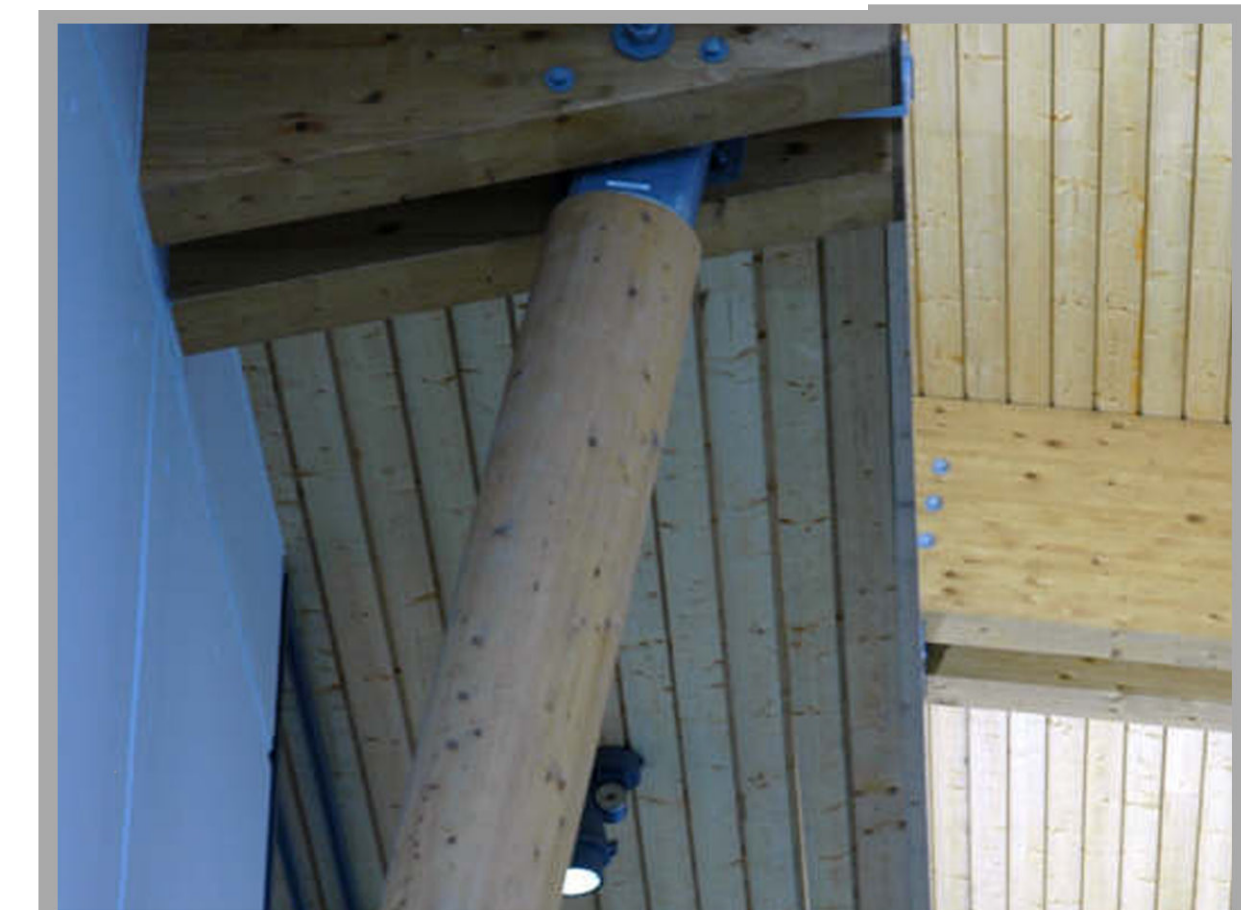
LAMINATED TIMBER COLUMNS
