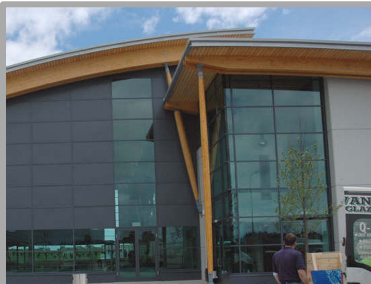
LAMINATED TIMBER COLUMNS
